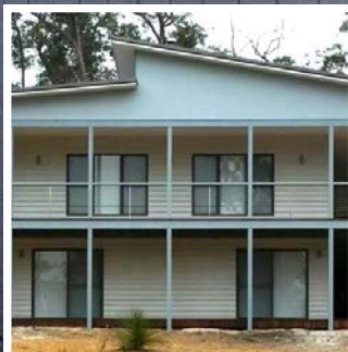
Weatherboards, fascia and exposed rafters
