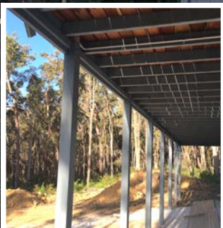
Subfloors, structures and decking posts
